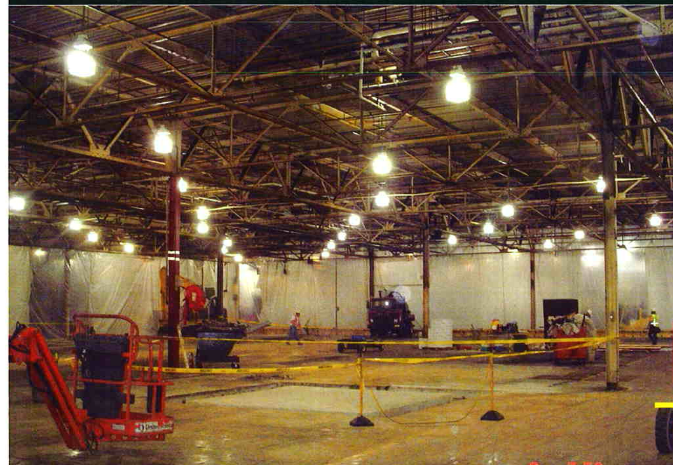
Courtyard Office – April 2005
