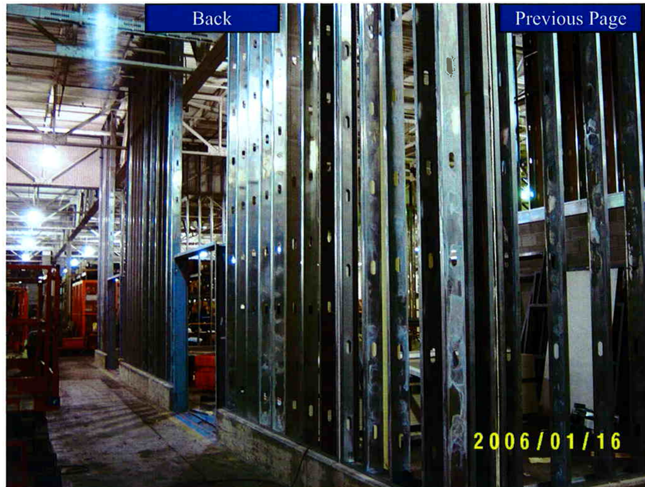
Camshaft Dept. – Demising Wall Construction
