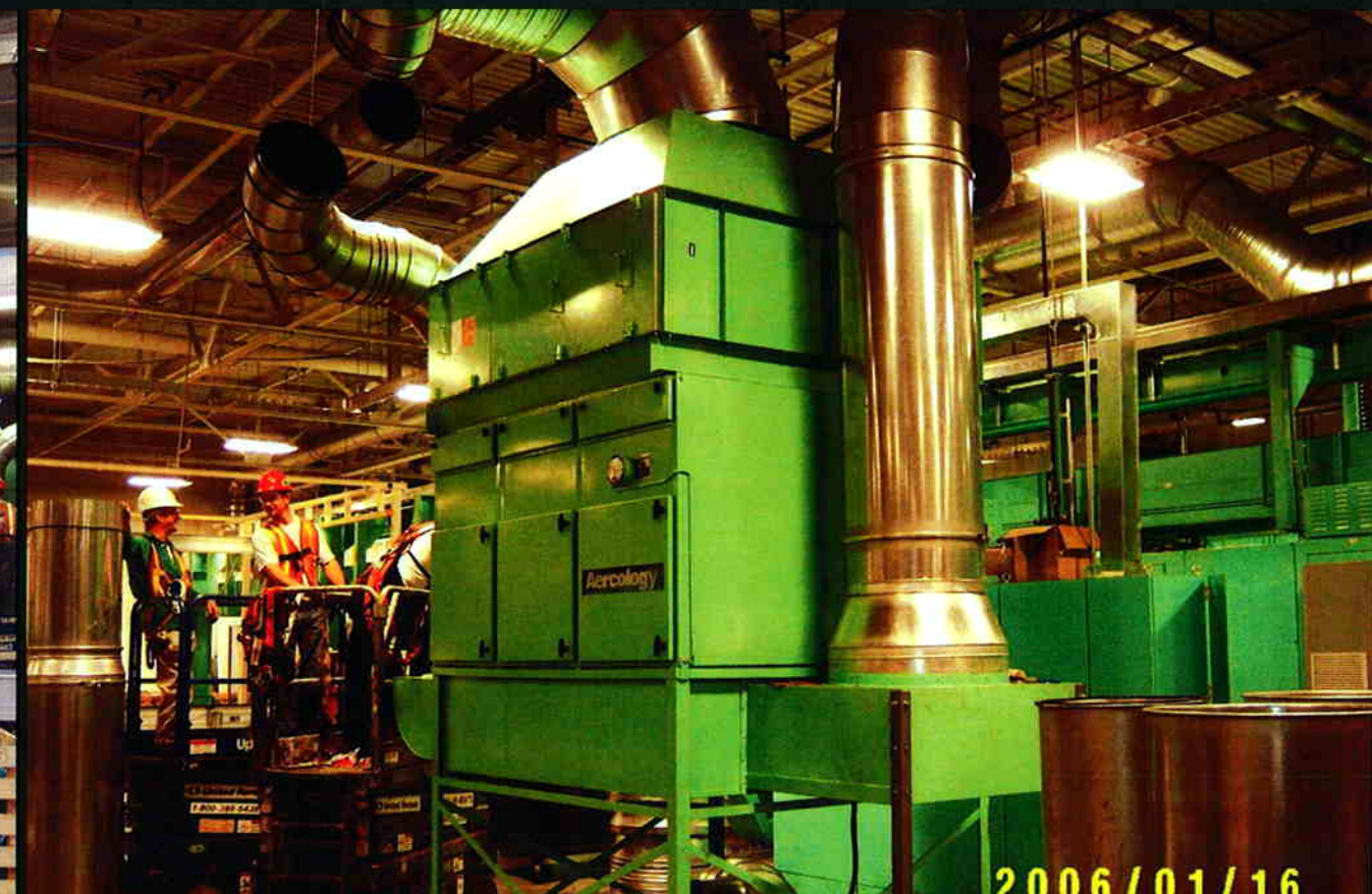
Crankshaft Dept. – New Aercology Unit Installation
